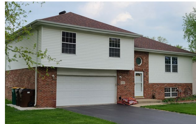
4 #4 9306 Pleasant (same side of block)- brick conforming
